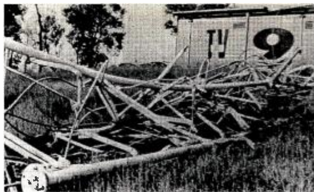
Tower tragedy. KCRG-TV Cedar Rapids was back on air with regular programming last Friday (Oct. 5), within 36 hours after its 2,000-foot tower at Walker, Iowa, collapsed, killing five workers and injuring several others. Working around clock, KCRG-TV Chief Engineer Walter Alliss Jr. and RCA field representatives moved and installed transmitting equipment at old station tower at Hiawatha, Iowa. (Story page 55.)
